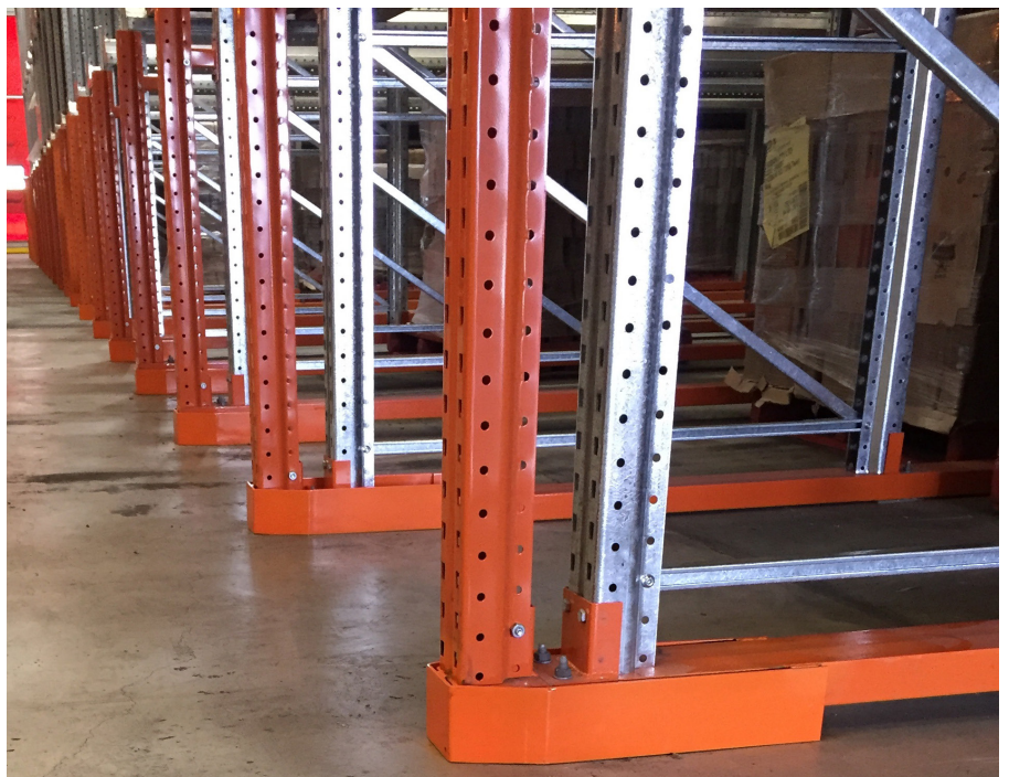
Bull-nose Protector eliminated gaps underneath the front of the channel.
